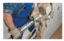
As a demolition tool, the DARDA HCS8 B replaces the sledge hammer as a very efficient tool that will precisely break through brick walls up to 32 cm (12,6 inches) thick.
