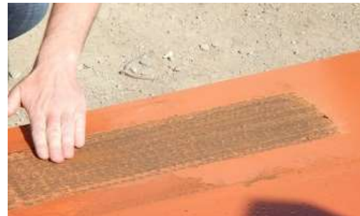
Painted steel surface
